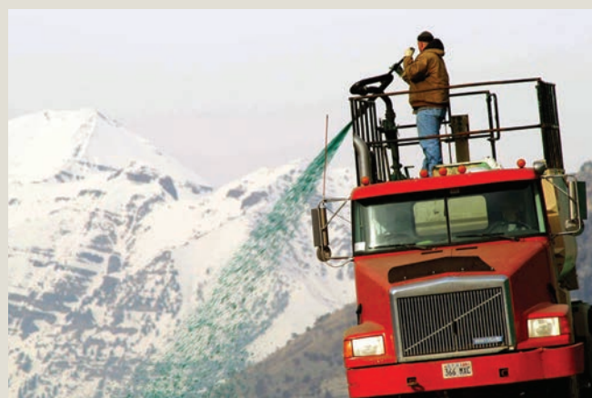
In hydraulic applications the hydromulch slurry may contain a variety of planting aids along with the seed, including fertilizer, mycorrhizal inoculant or tackifier. ©Ryan Timoney/Granite Seed Company
